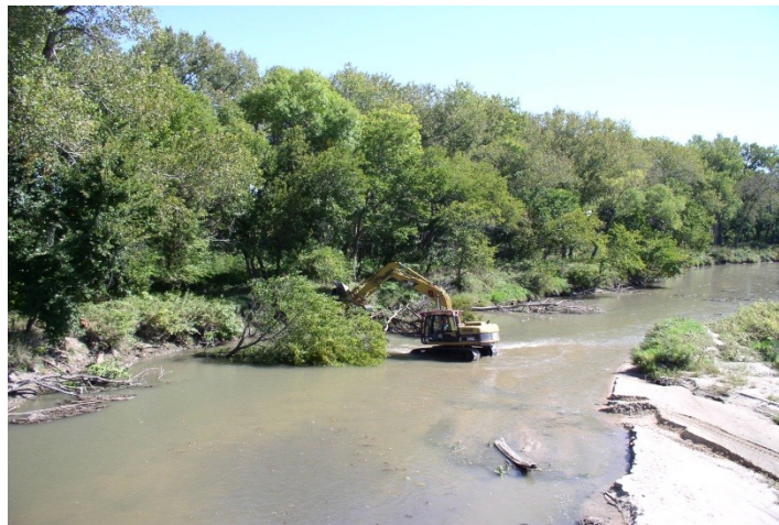
Pictured above is tree shearing along the river by Frahm Construction.
